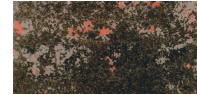
Wa 2 Thorough high-pressure water blasting
