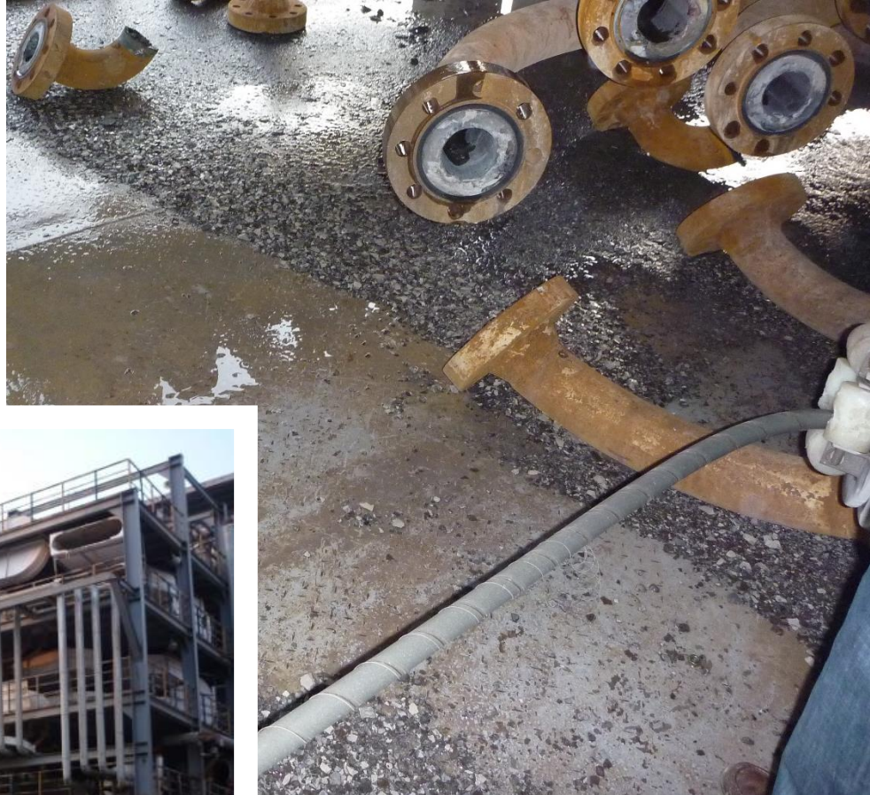
Pipe work cleaning with a rotating hose reel
